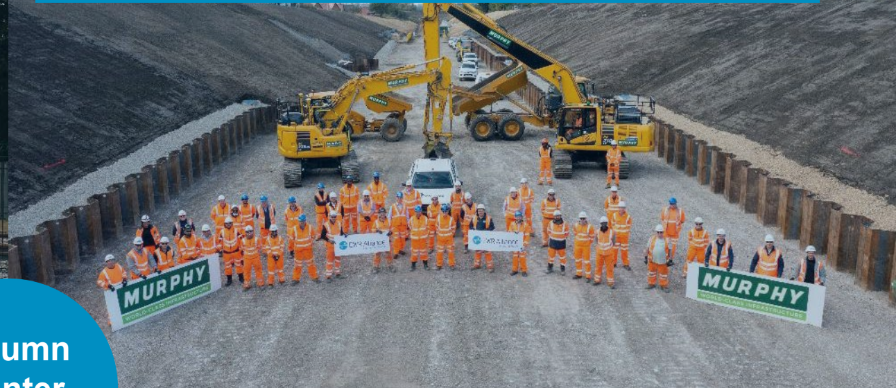
Earthworks Sectional Completions – September 2021 onwards
