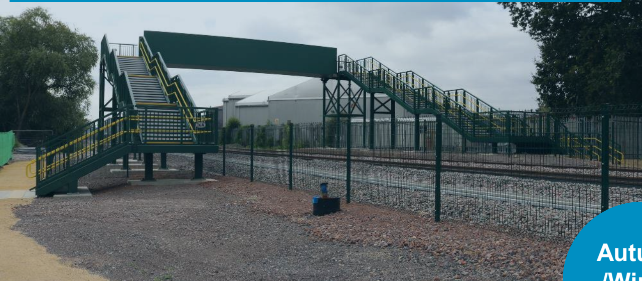
OXD36A Jarvis Lane Footbridge handover – first of five new footbridges to be completed – September 2021
