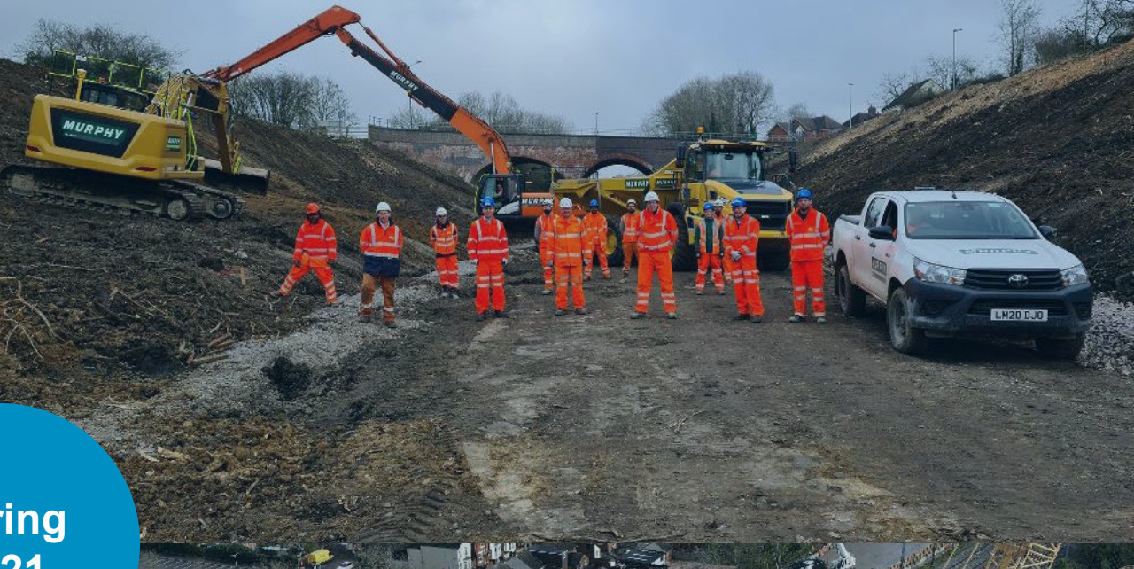
Main Earthworks Start on site – March 2021
