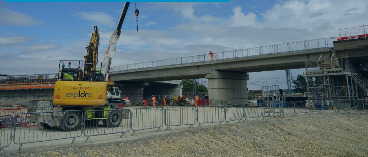
All spans completed at Bletchley Flyover – August 2021
